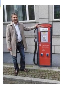
The 'Strom Tankstelle' or 'Electricity pump' is a CP installed with two dedicated EV parking places, and further two for e-bikes, on the forecourt of the Sparkasse (Savings bank) office building. They are very simple charging points, with a 220 Volt plug, designed to be highly visible to support early EV adopters. The CP draws on renewable hydro electric energy from the Main River.
